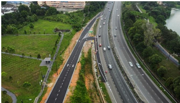
Junction to burial grounds via MRR2 towards Batu Caves
